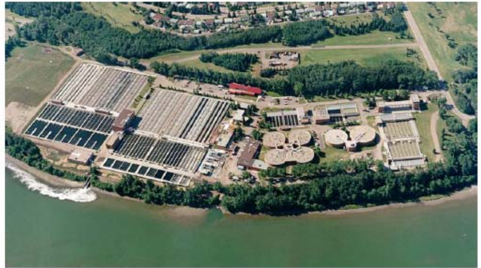
Gold Bar WWTP
