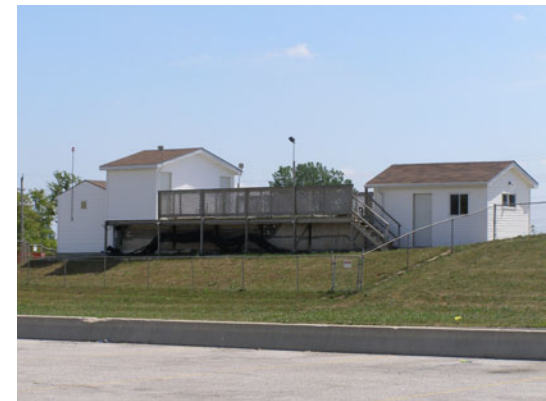
5 th Wheel Truck Stop WWTP – Dorchester, ON – 45m 3 /day SBR
