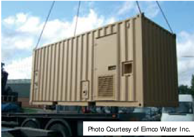
PACKAGE PLANT (usually up to 200m 3 /day) Steel or Pre-cast Tanks
