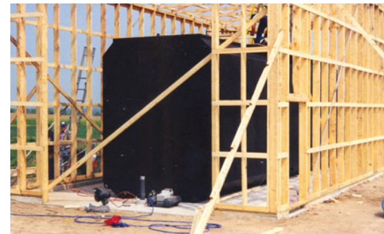
Sentinel WWTP – 33m 3 /day SBR Photos Courtesy of Fluidyne
