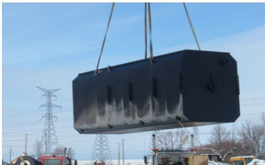
Sentinel WWTP – 33m 3 /day SBR Photos Courtesy of Fluidyne
