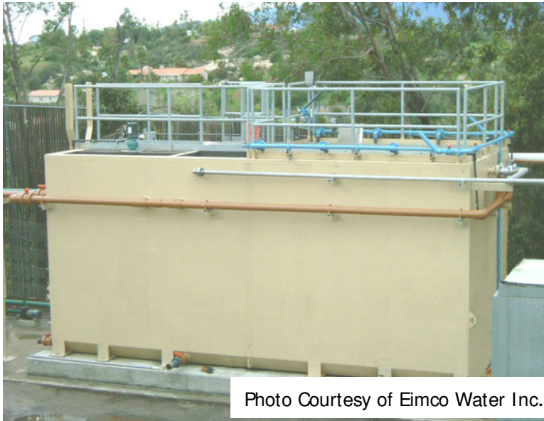
PACKAGE PLANT (usually up to 200m 3 /day) Steel or Pre-cast Tanks
