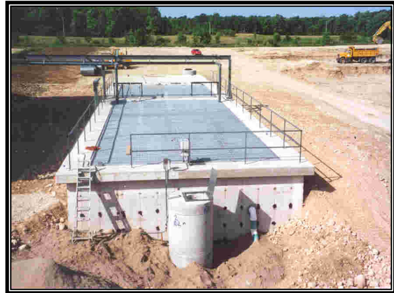
PRE-ENGINEERED PLANT (usually up to 3800m 3 /day) Poured In Place Concrete Tanks
